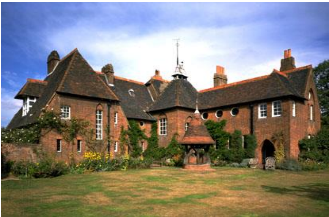
Philip Webb, Red House, Bexleyheath, U.K. (1859). Gothic flavor and spirit without any discernable style; historical, yet structurally modern.
