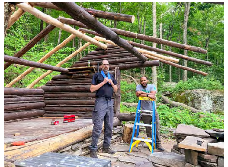
Volunteers Charles Whitaker and Demetrius Watson frame the Baldwin Memorial Shelter roof.
