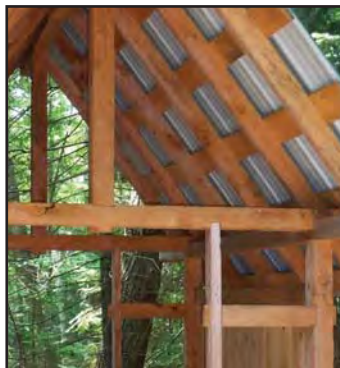
Post and Beam
